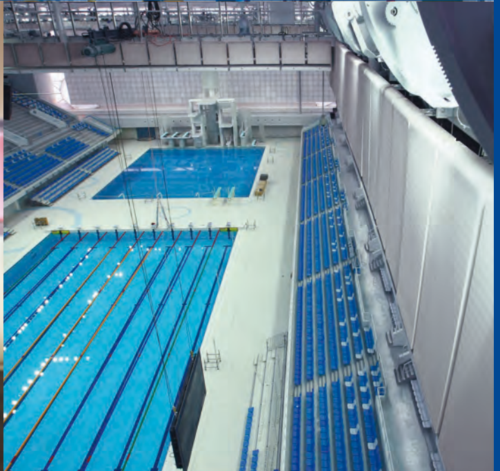
Soundproofing at the National Aquatics Center in Beijing, CN
